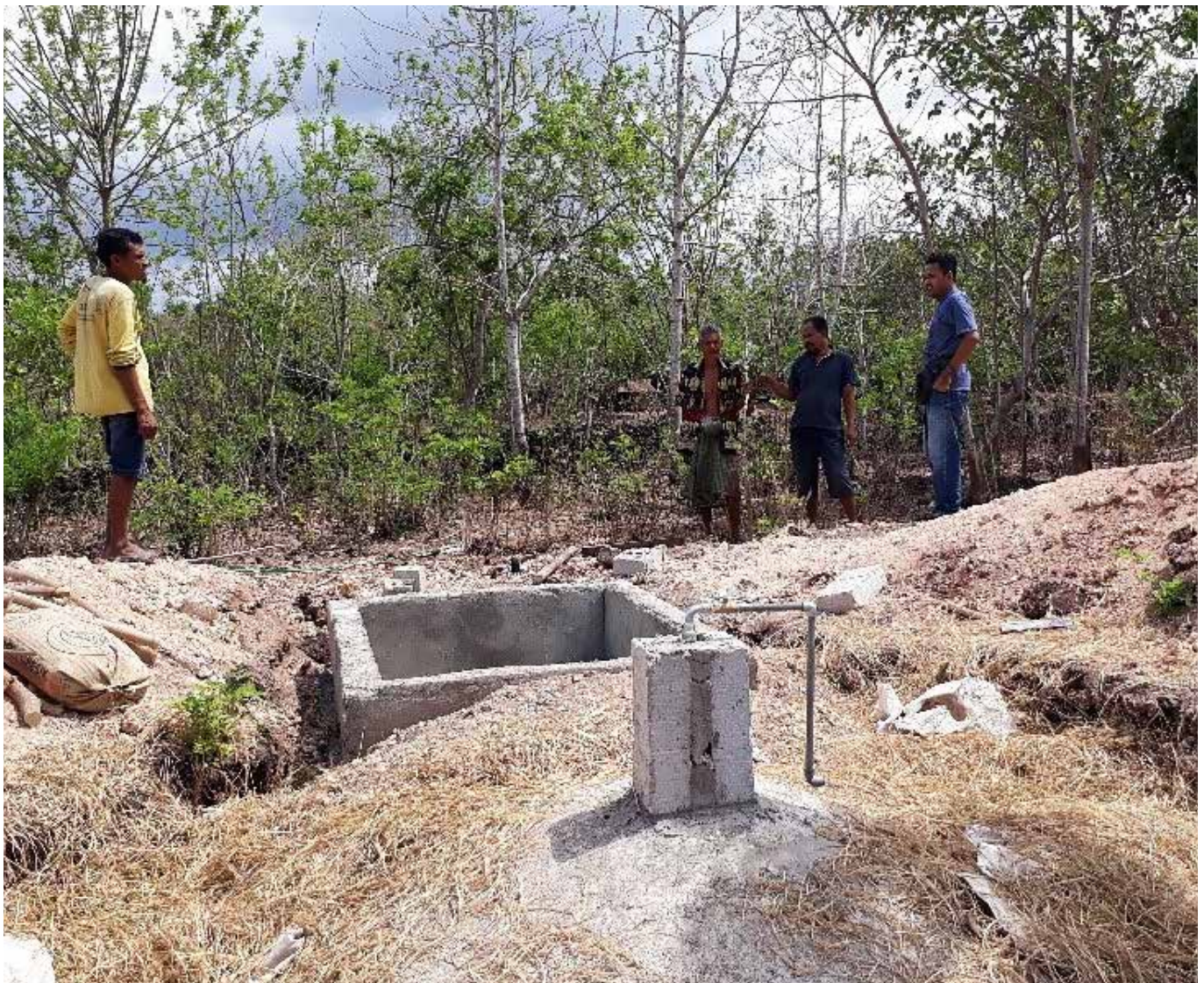
Quality inspection on biodigester in Kataka village of East Sumba
